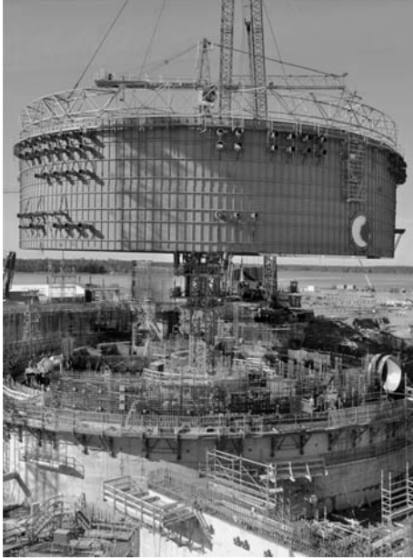
Fig. 4.20 OL3, lifting in the liner ring [22]
