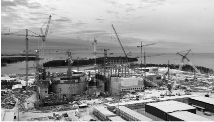
Fig. 4.14 OL3, cranes used on nuclear island – reactor building and auxiliary buildings (left) and conventional island (right) [22]
