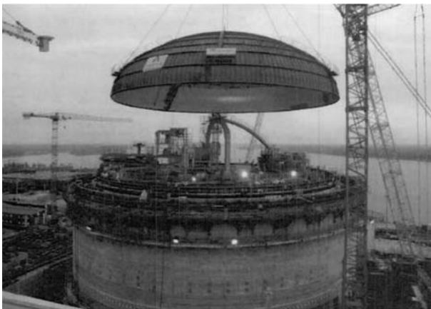
Fig. 4.21 OL3, lifting in the liner dome [30]
