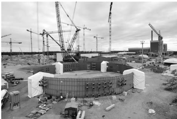
Fig. 4.19 OL3, Assembling the steel liner on site [22]
